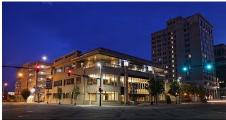
Kansas Leadership Center and Kansas Health Foundation Conference Center.
