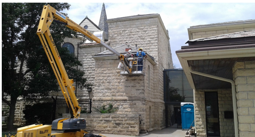
Guttering being replaced on the church.
