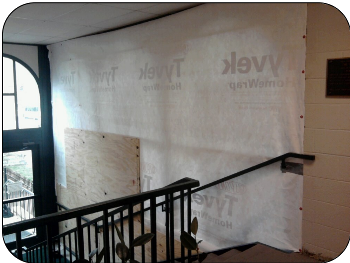
Framework securely covered before replacing glass panels on west side of Ed. Bldg. A construction lift waits outside.
