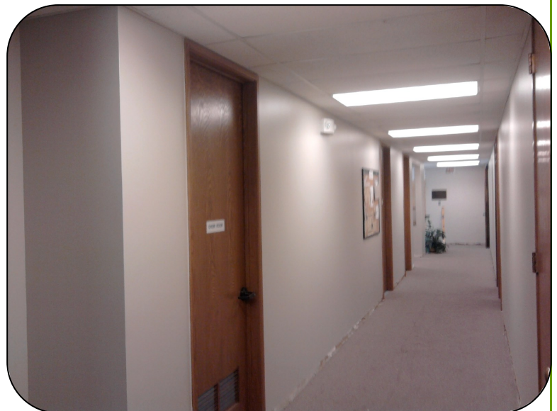
New paint & lights brighten the hallway; the atrium in progress
