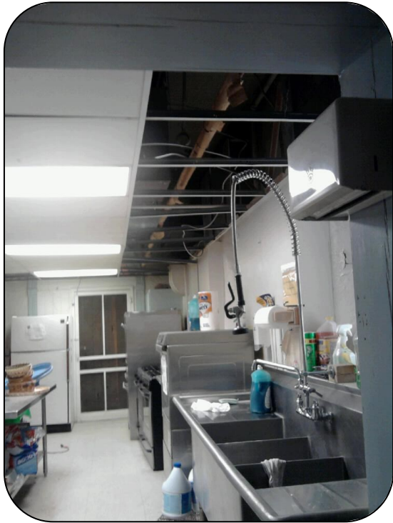
Wires & pipes exposed in undercroft kitchen
