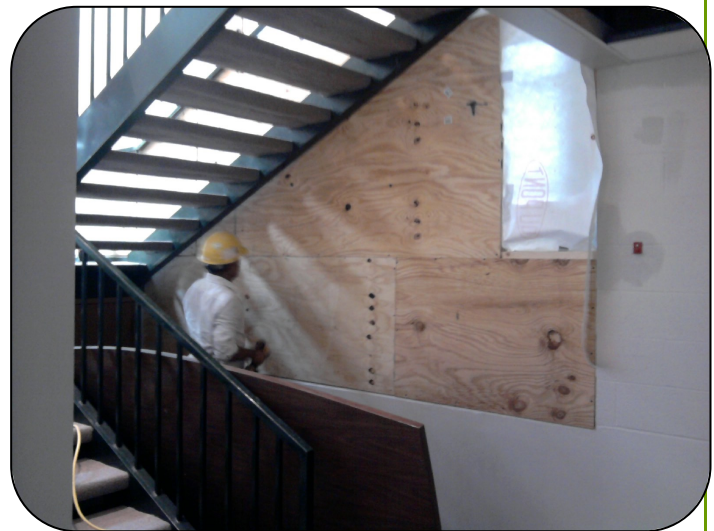
Framework securely covered before replacing glass panels on west side of Ed. Bldg. A construction lift waits outside.
